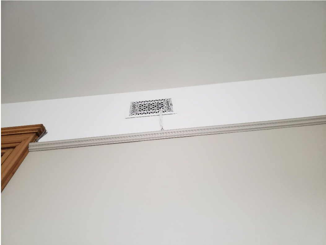
Figure 3: Cable Installation in Wall Vents
