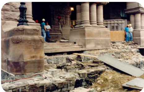
Extensive restoration of the exterior masonry and major modifications to the main entrance in the 1990s. As sandstone is a soft stone, it erodes very quickly.
